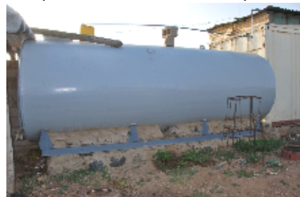
(Bar Sinit – Cisterna –2011)
